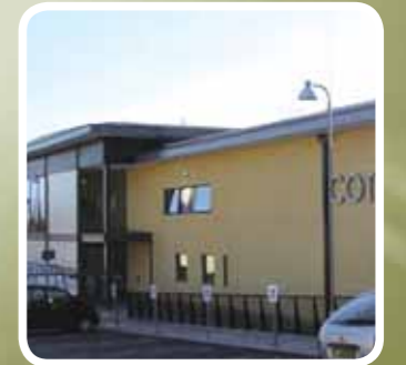
A 286kVA Powerstar unit is installed at the council owned Cotswold Leisure Centre
